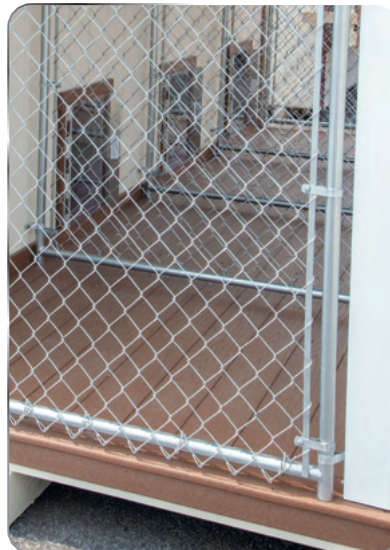
COMPOSITE DECKING ON RUNS
